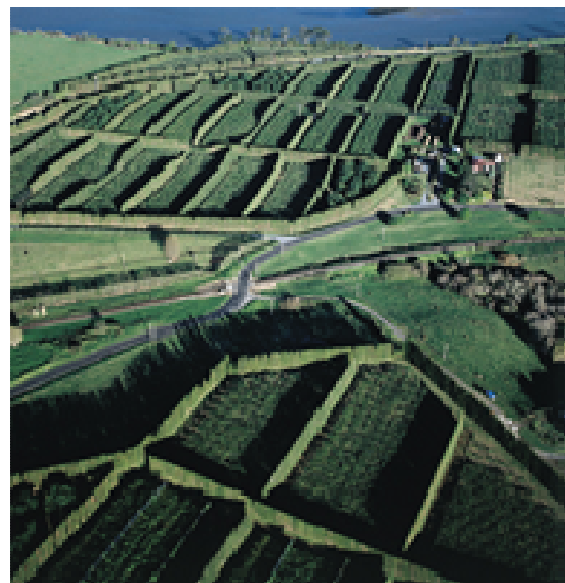
Figure 1. Shelterbelts in kiwifruit orchards – a conspicuous feature of the Bay of Plenty landscape.
